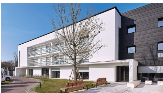
IT Elderly House "Ca' dei Fiori" https://int.baumit.com/lifechallenge2020/projects/thermal-renovation/2632/1
