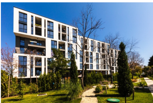
BG Atlantis Residence Park https://int.baumit.com/lifechallenge2020/projects/multi-family-residential/2454/1
